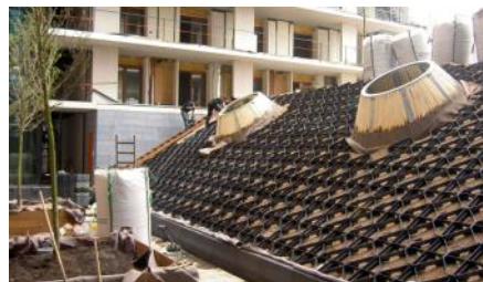
Two layers of Georaster® filled with substrate ensure proper supply of water and nutrients for the lawn.
