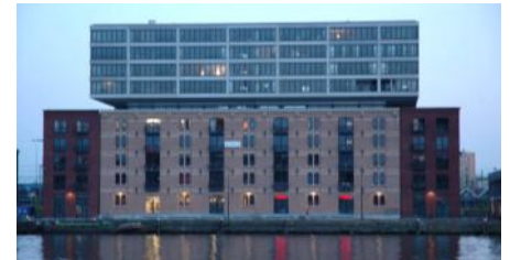
View from the Java island to the former warehouse.
