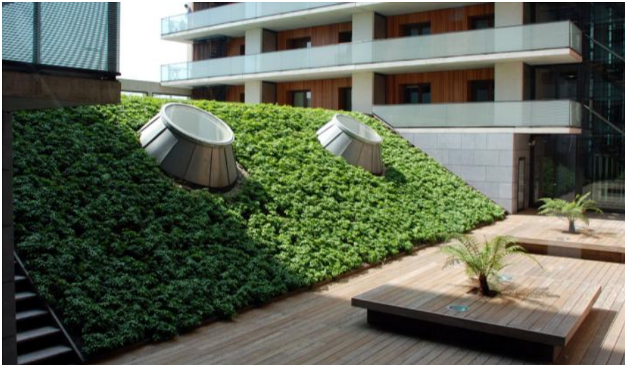
The inner courtyard of the "Australiëgebouw" with Pitched and Flat Green Roof.
