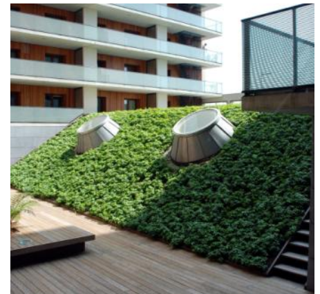
The maintenance of the lawn turned out to be costly. Therefore it was exchanged by a low maintenance ground cover planting.
