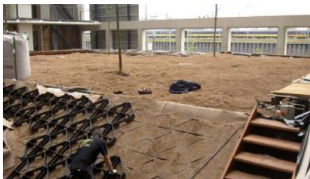
The proposed turf was intended to invisibly connect the pitched roof area to the flat roof area.
